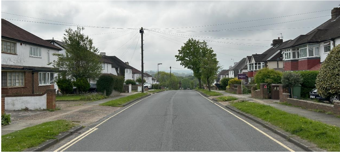
Figure 7 – Roof Lines following the natural incline on Newbury Gardens down to Stoneleigh Park Road
